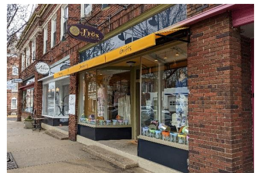
Awnings, window lettering, signage create inviting storefronts.
